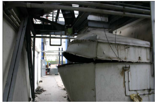
Catalytic oxidizer, after explosion
